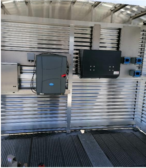
Online gauges inside climate shield
