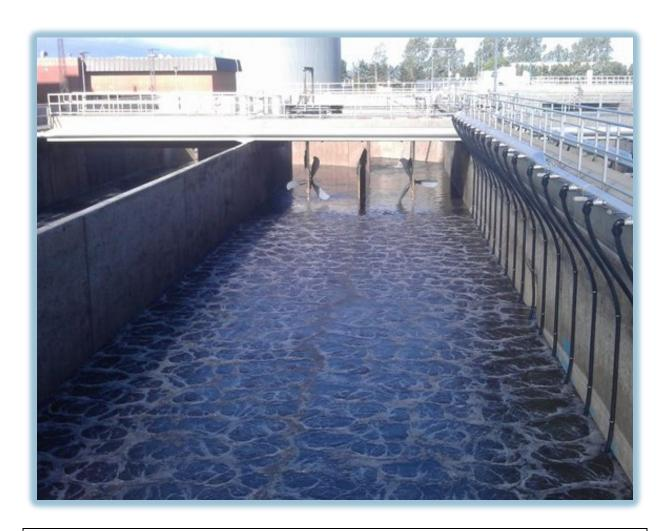
**Task:** Nyt beluftnings system på Renseanlæg Aalborg Øst, omfattende blæsere, flowdanner distributionsrør, stribe diffusorer mv. (Aalborg Øst har en kapacitet på (95.000PE) New aeration system at wastewater treatment plant Aalborg Øst, including fans, flow forming distribution pipes, stripe diffusers, etc. (Aalborg Øst has a capacity of (95.000PE))
